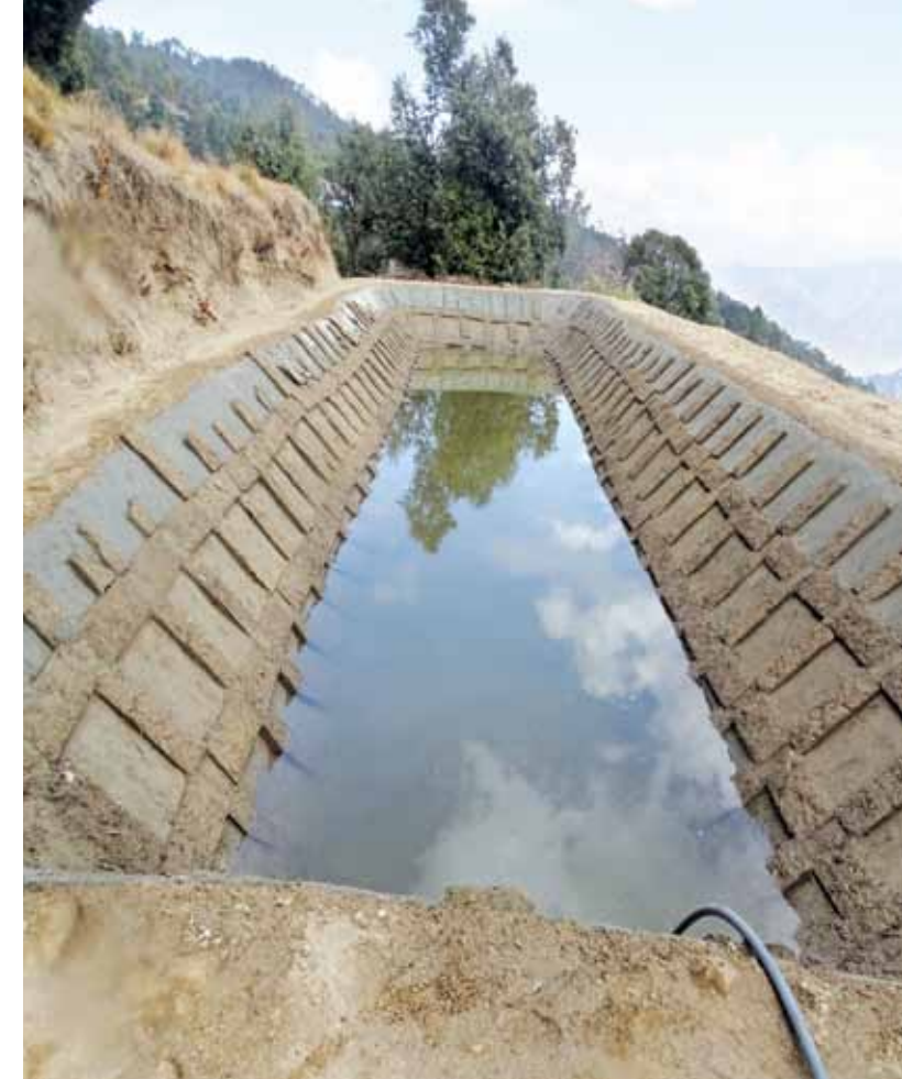
Poly cement tank – A low cost option for water harvesting
