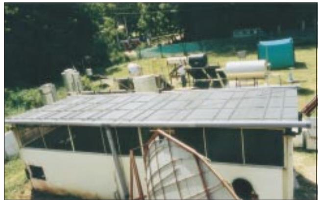
Roof integrated unglazed solar-air heater. This costs around Rs 1,000/m<sup>2</sup>. Its single module evaluation recorded a temperature rise of 15°C.
