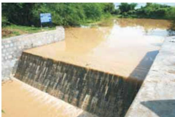
Check dam constructed under the project, Mirzapur
