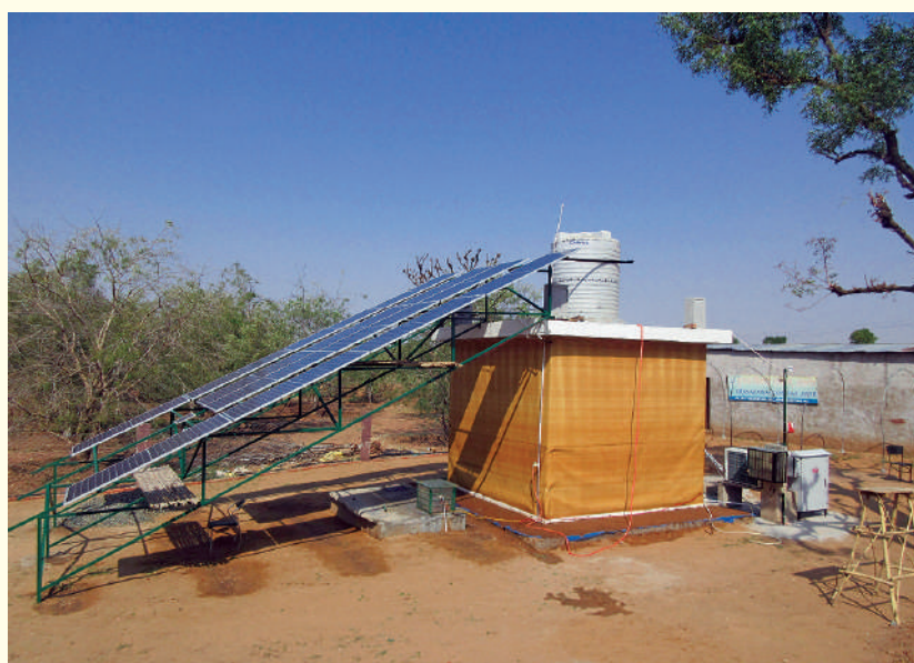
The newly operational gridless, batteryless solar Pusa-FSF at village Picholiya, Ajmer, Rajasthan
