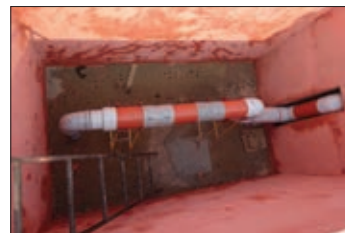
Filter assembly of drainage-cum-recharge structure (Pusa)
