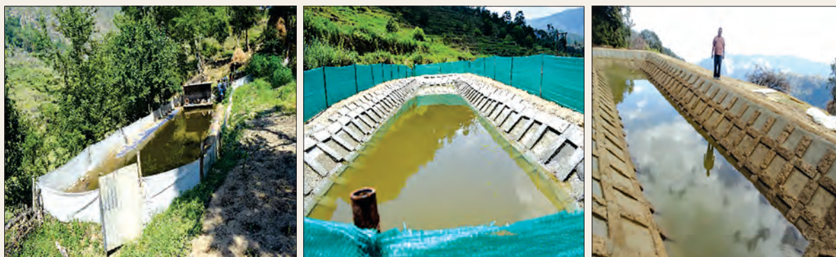
Poly cement tank at farmer's field
