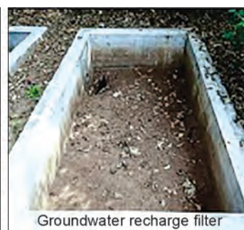
One stage downward flow recharge filter
