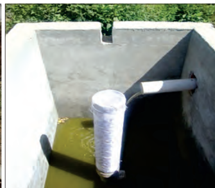
Recharge cavity well
