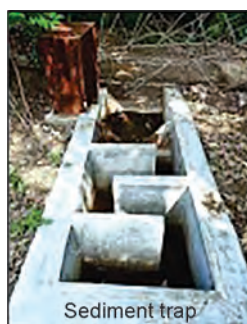
One stage downward flow recharge filter
