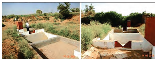
One stage upward flow recharge filter
