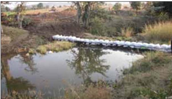
Low cost sand bag check for enhancing surface water storage and sub-surface flow to adjoining farm ponds
