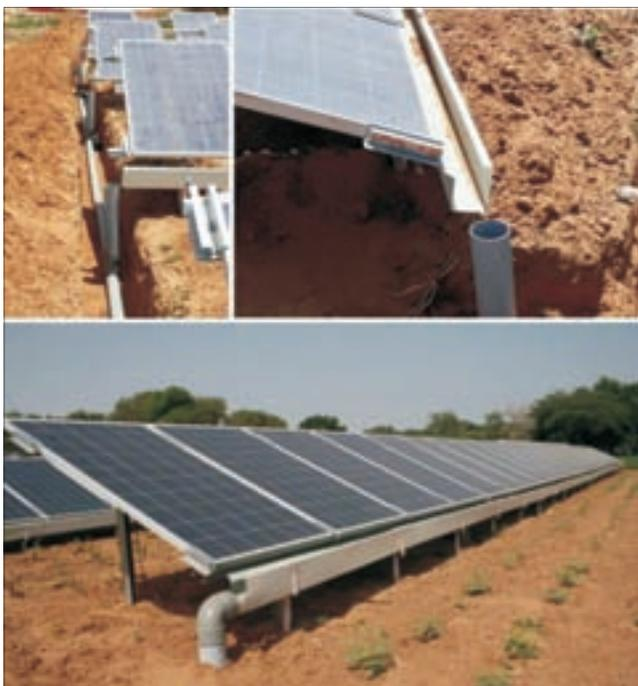
Fig. 5 Rain water harvesting system from top surface of PV module
