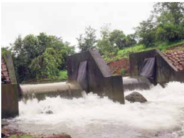
A flexible rubber dam for water harvesting in watershed
