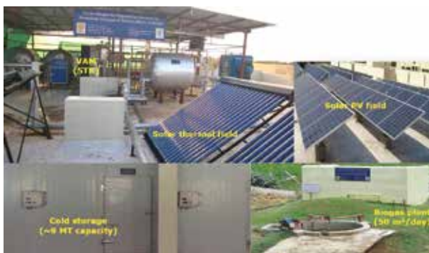
Solar refrigeration & PV power facility
